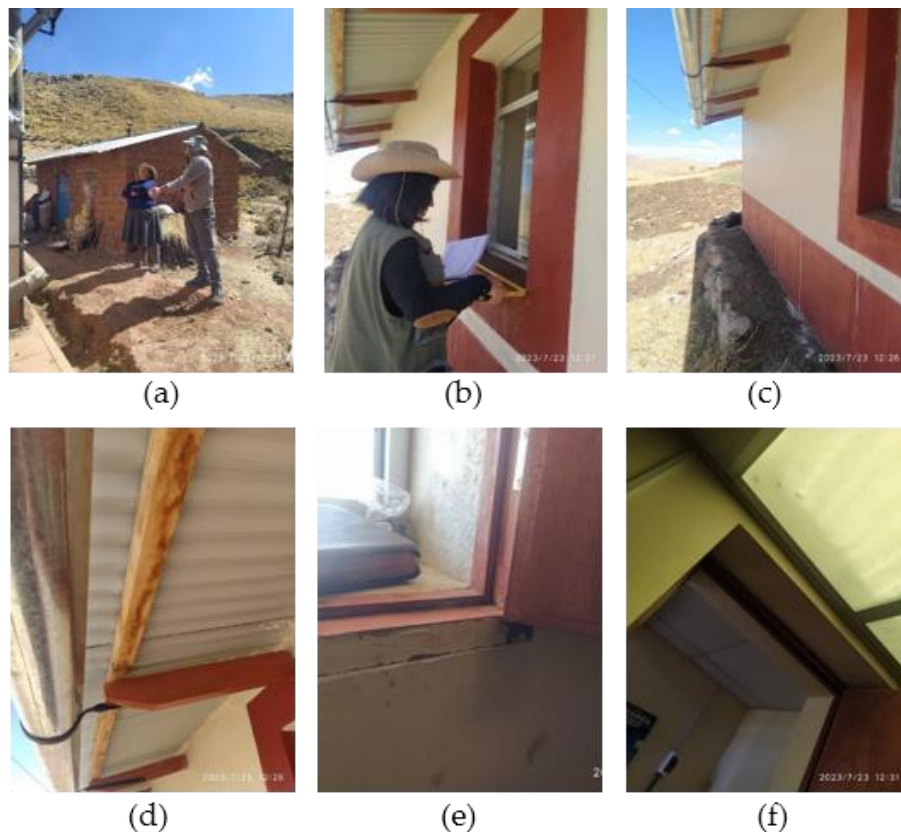
Figure 7: Photographic record of construction materials verification. (1) Interview with the homeowner. (2) Verification of measurements. (3) State of repair of the foundation, subfloor, and wall of the home. (4) Detail of the roof overhang. (5) Detail of the aluminum window frame and wooden shutter. (6) Detail of the polycarbonate skylight in the social area inside the home.
